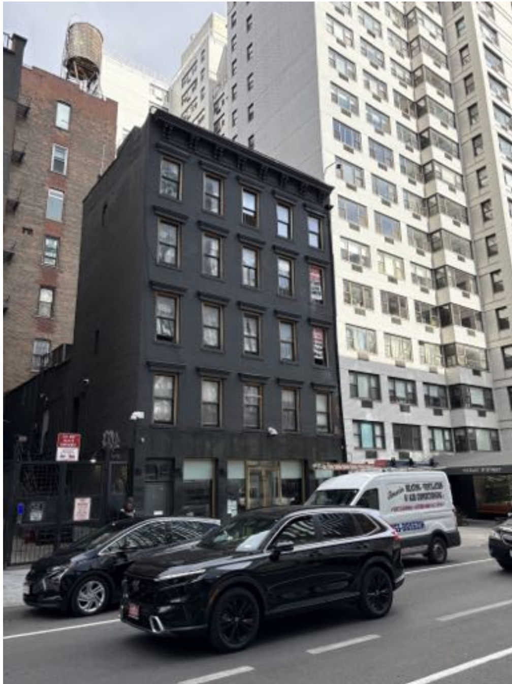
Figure 8: Front and west facades as observed on November 7, 2025. The exterior configuration is structurally identical to that seen in figures 5 and 6.
