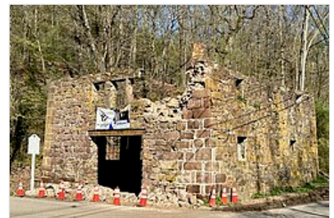
Damage to John Taylor's Grist Mill
